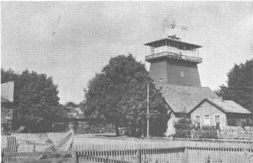
Water Tower, N.W. First and Adams
